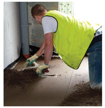
moisture contained in the mix. It is important to keep moisture content to the minimum as an excessively wet mix can result in shrinkage during curing, leading to cracking of the screed. However, too little moisture will result in unhydrated cement and therefore weaker screeds, so a balance must be struck.
